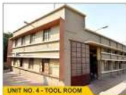
UNIT NO. 4 - TOOL ROOM
