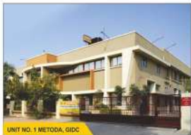
UNIT NO. 1 METODA, GIDC
