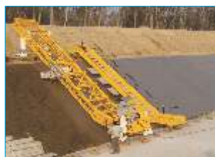
Concrete Canal Paver
