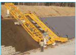
Concrete Canal Paver
